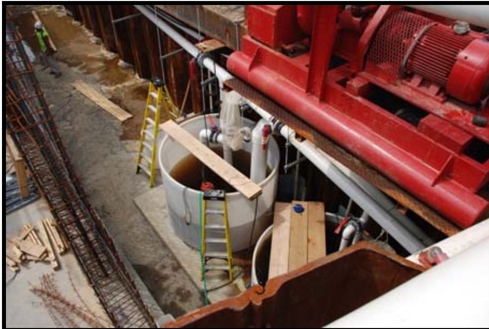
Figure 4. The intake (top) and control sample tanks viewed from the support platform.
